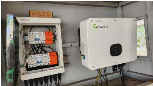
Gambar 3. Panel DC Combiner dan Inverter On-grid.
